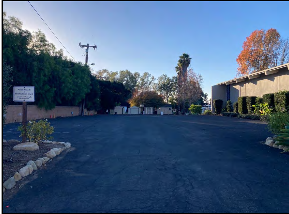
Photo 1: View of Christ Lutheran Church parking lot entrance from Covington Way (Aspect: South).
